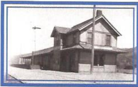
The Depot is a standard 22R design with offices on the right, freight shed on the left, and living quarters above.
